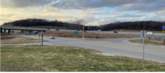
Facing Northwest on Donahoo Rd, Subject Property on Northeast (right) corner of I-435 On Ramp
