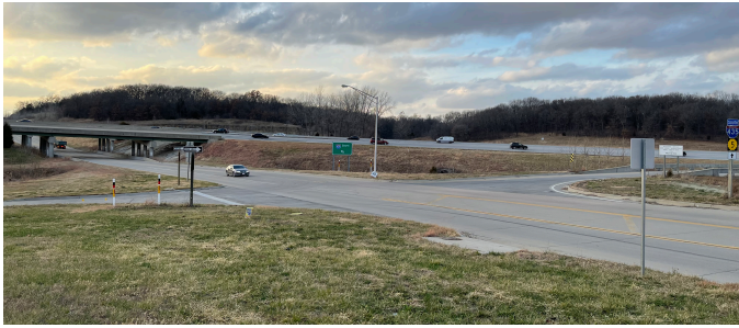
Facing Northwest on Donahoo Rd, Subject Property on Northeast (right) corner of I-435 On Ramp
