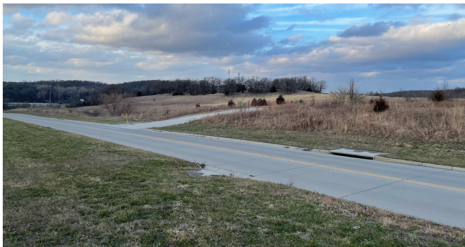
Looking Northwest; South Property Line Donahoo Access Rd
