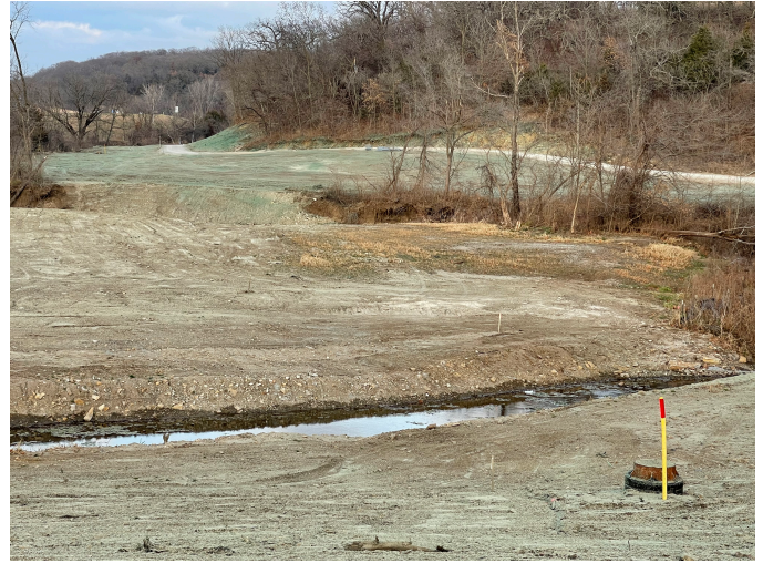
Looking North; West Property Line, Connor Creek & Sewer Line
